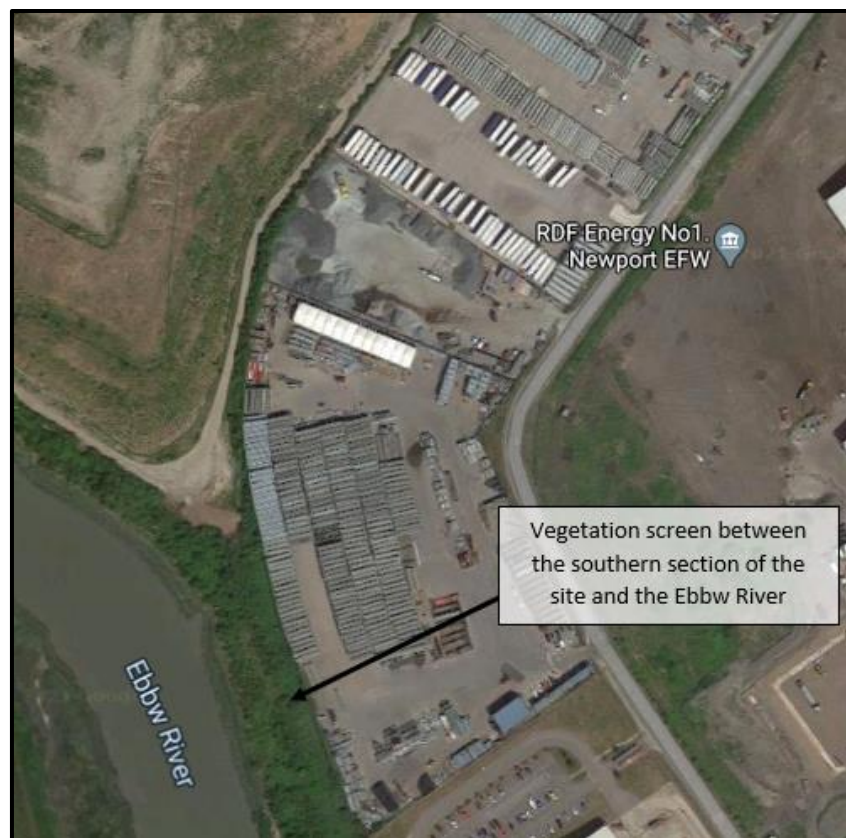
Figure 6: Satellite image of the site indicating the presence of the vegetation screen between the western boundary of the application site and the Ebbw River as required by application ref. 07/0592
